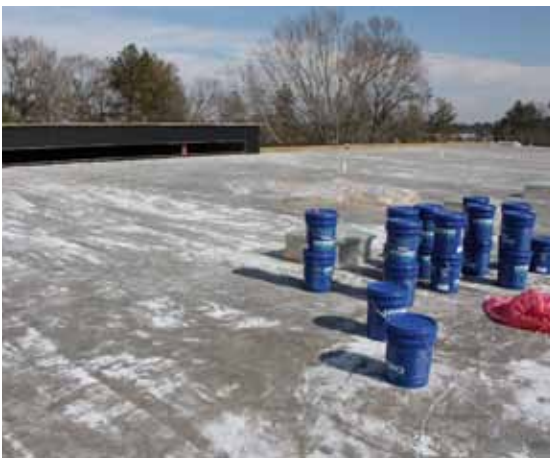
Applying BarrierGuard slurry
