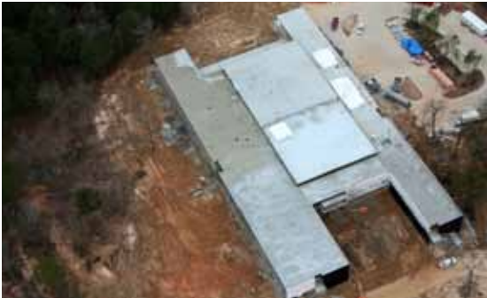
Applying BarrierGuard slurry
