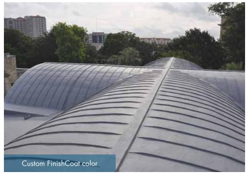
A fluid-applied product, the PremiumCoat® System was an ideal choice for the unique shape and structure of the Alamo Shrine roof; in a sense, PremiumCoat® acted as a "custom fit" product, completely adhering to every curve while maintaining the historic "character" of the metal panels. To preserve the historic appearance of the roof, a custom FinishCoat color was tinted to match the color of the aged metal panels. Officially named Dover Grey, the color was nicknamed "Alamo Grey" on site.
