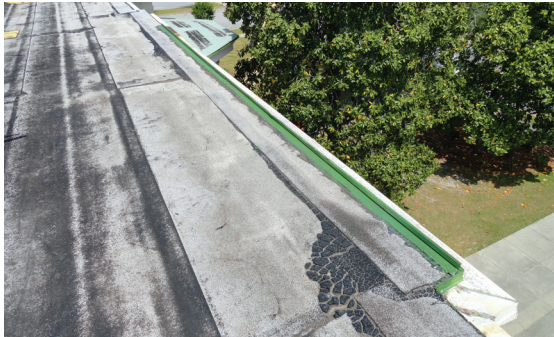
Existing modified bitumen roof
