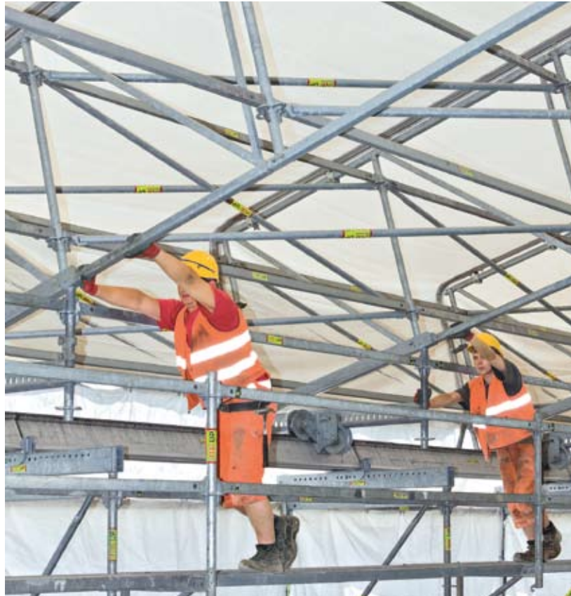
LGS roofs can easily be moved by hand and are also equipped with brakes, ensuring a fast moving procedure. Photo Credit: PERI GmbH.
