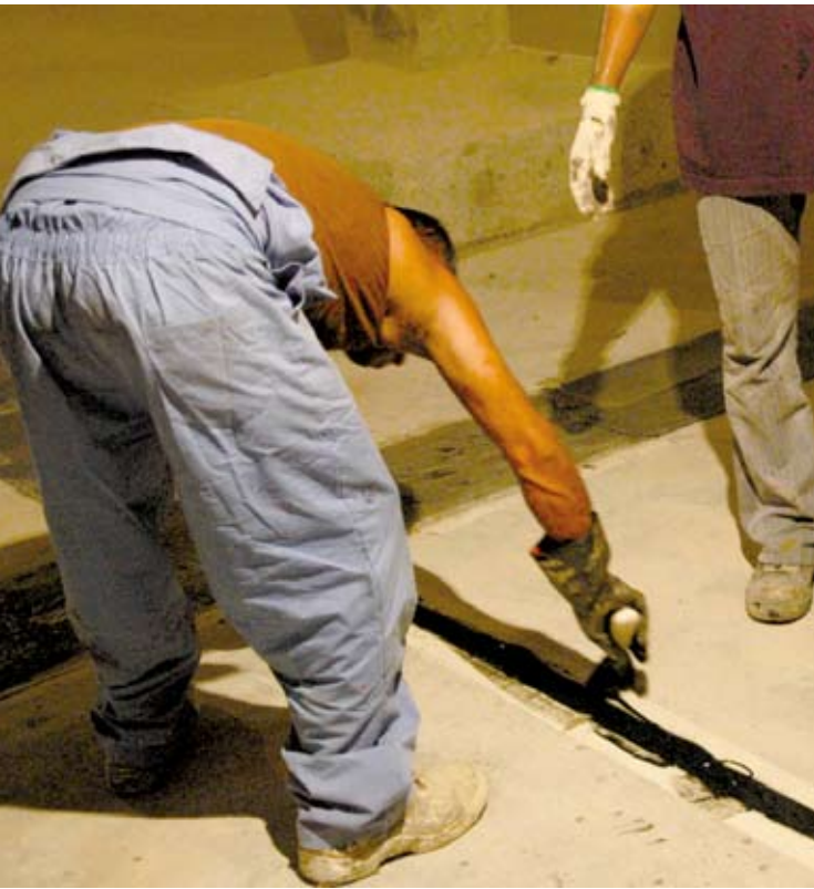
Mastic application in the joints.
