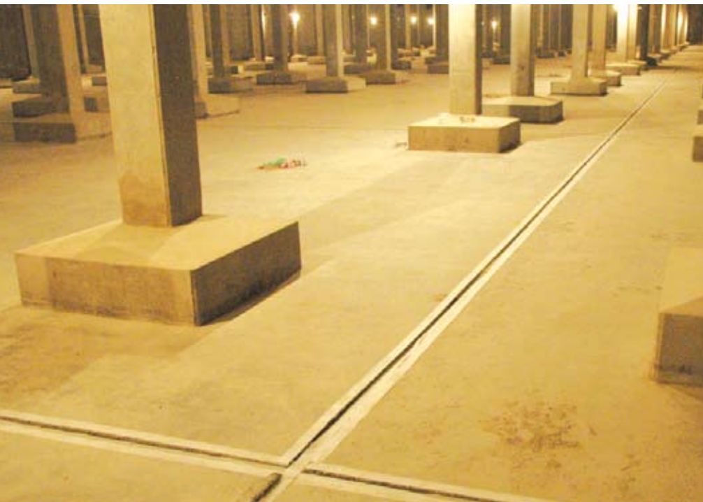
Before applying Elastuff 120.
