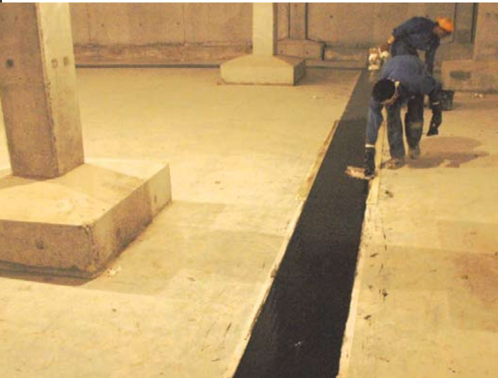
Membrane waterproofing application.
