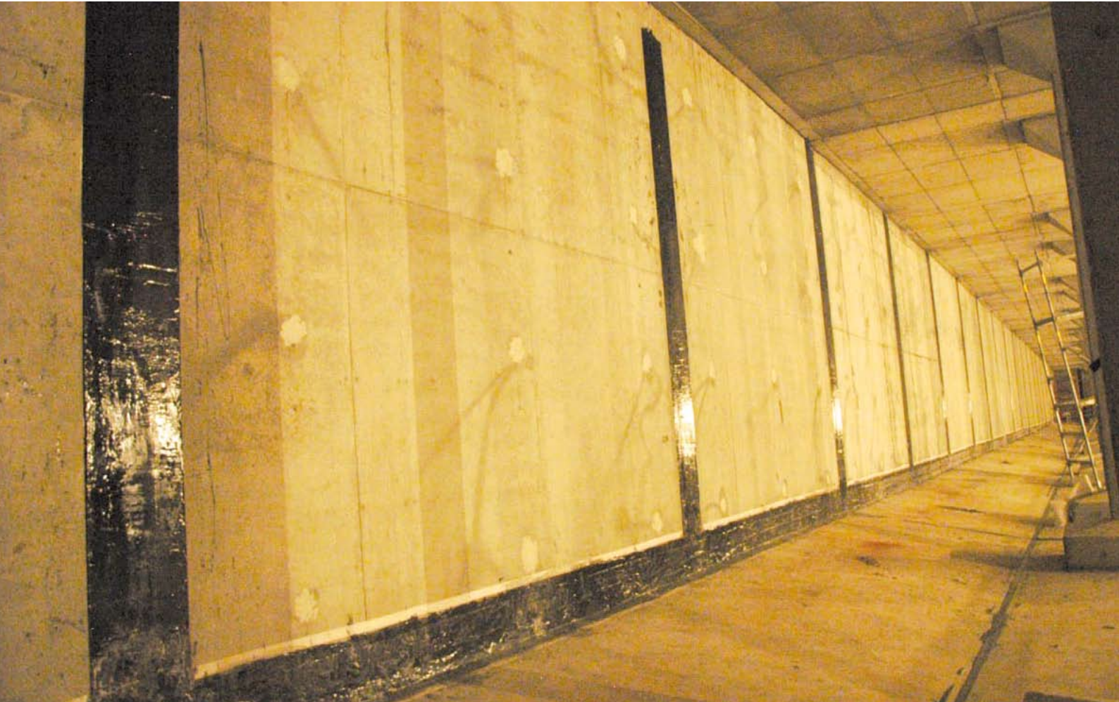
Wall waterproofing application.
