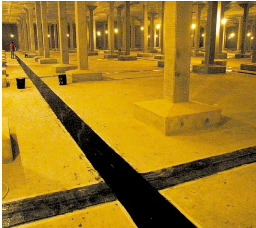
Overall waterproofing application.
